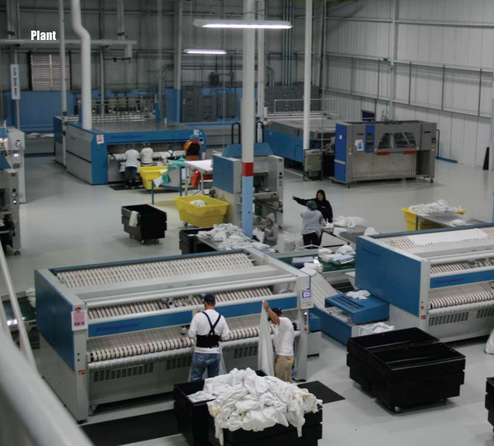
Employees feed flatwork on the finishing side of Reino Linen Service's 92,000 square-foot healthcare plant that opened last July in Brownstown, MI.
